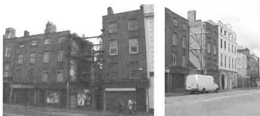
Figure 5 – Before and after images of a building clean up.
