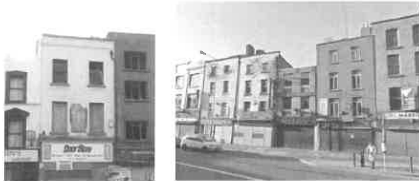
Figure 4 -- Thomas Street Derelict Buildings
