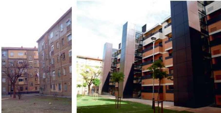
Fig 4. Public green zone and towers of installations
